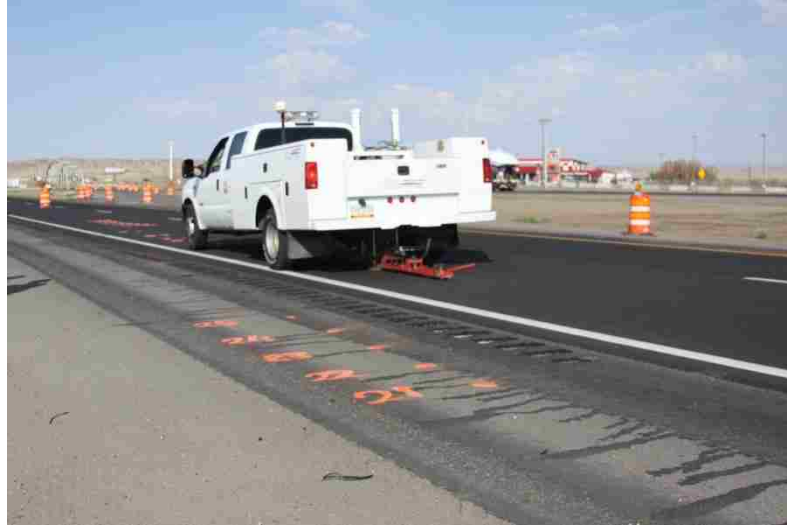
Figure 41. Conduction of FWD test on I-40 pavement
