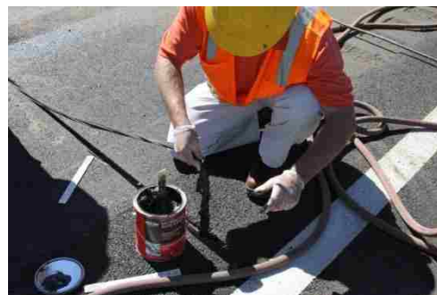
Figure 24. Installation of temperature probes
